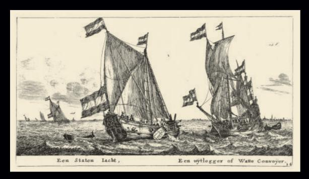
A States Yacht and a *Wadconvooier*, etching by Reinier Nooms (1623-1664). In this etching Nooms shows the difference between a States yacht and a *wadconvooier*. States yachts were luxury vessels; the *wadconvooier* was a small armed boat, designed to protect inland boats against enemy warships and privateers. The boat is gaff-rigged and has a small mizzen mast.
