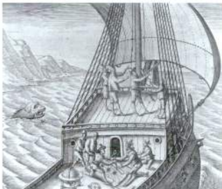
View of a ship's deck with a marine astrolabe and globe. Sailors are working on a chart with pair of compasses and a ruler. Another is at the foredeck measuring height with a cross staff (cross staff). In his right is a man holding a quadrant.
